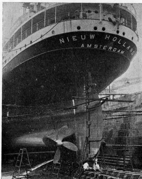
Measuring the rudderpintle clearance.
